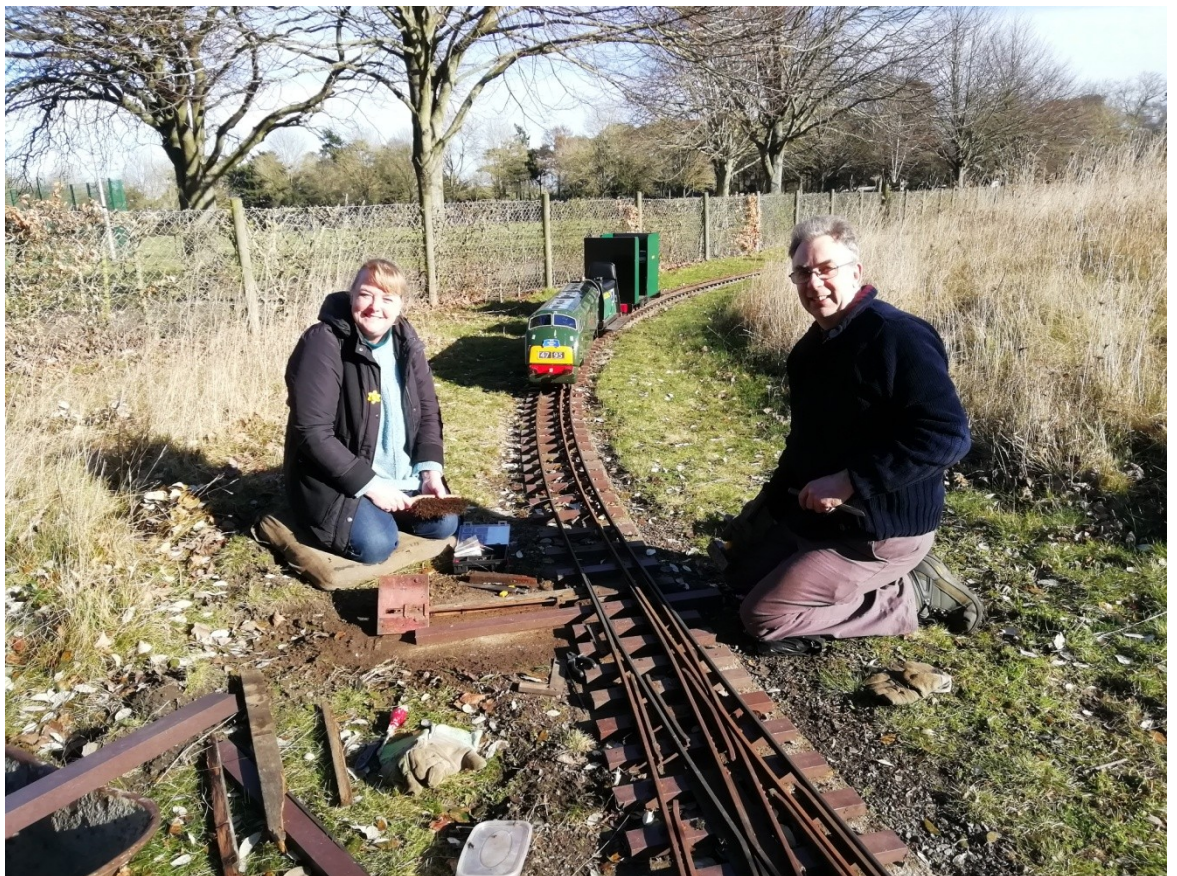
The third of the four points in the field being resleepered in plastic
